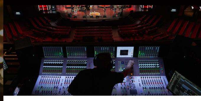
In January 2025, the Grand Ole Opry deployed a 62 fader Studer Vista X broadcast console, replacing a Vista 9 that had served them loyally for over a decade. This followed a 2024 upgrade of the front-of-house desk to a Studer Vista V, establishing full alignment between live and broadcast operations. The existing Vista 9 was repurposed and installed at the Ryman Auditorium.
